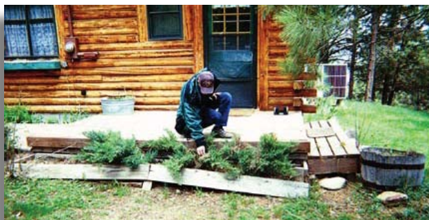
Flammable vegetation in direct contact with house
